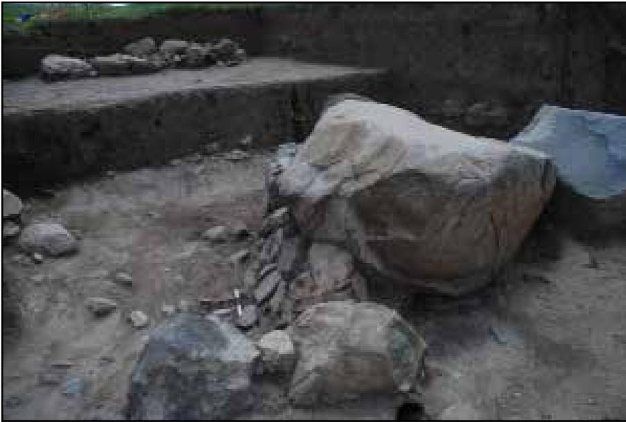
Fig. 4 – Area A: detail of the corner stone block of the wall and foundation substructure. From the northeast.
