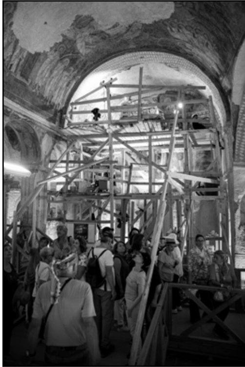
Figure 7. New Tokalı Kilise, south side. The scaffolding of the restoration worksite
