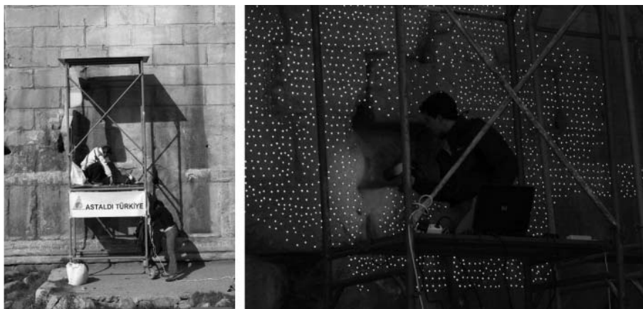
Fig. 12: The scaffold used to place the markers and a suggestive image of the markers
