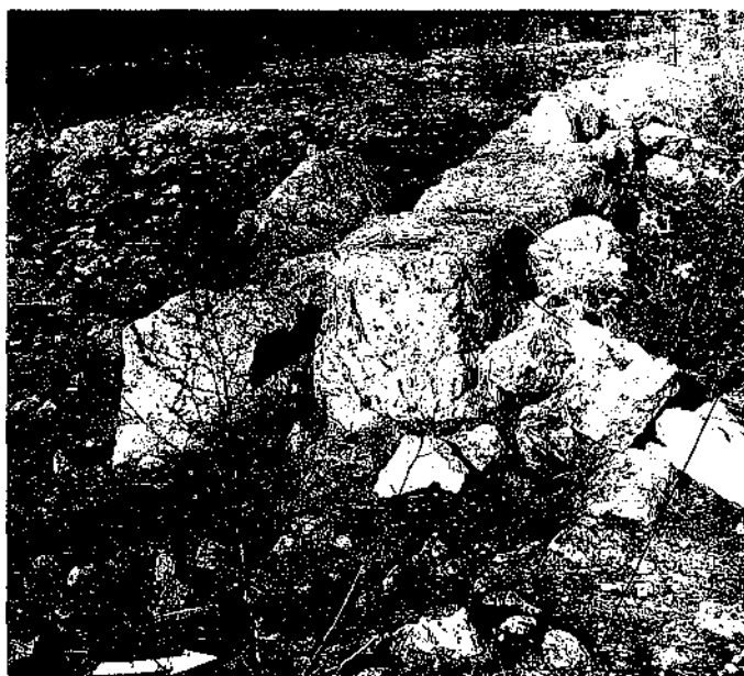
Fig. 14: SU 3, South-Wall from East.
