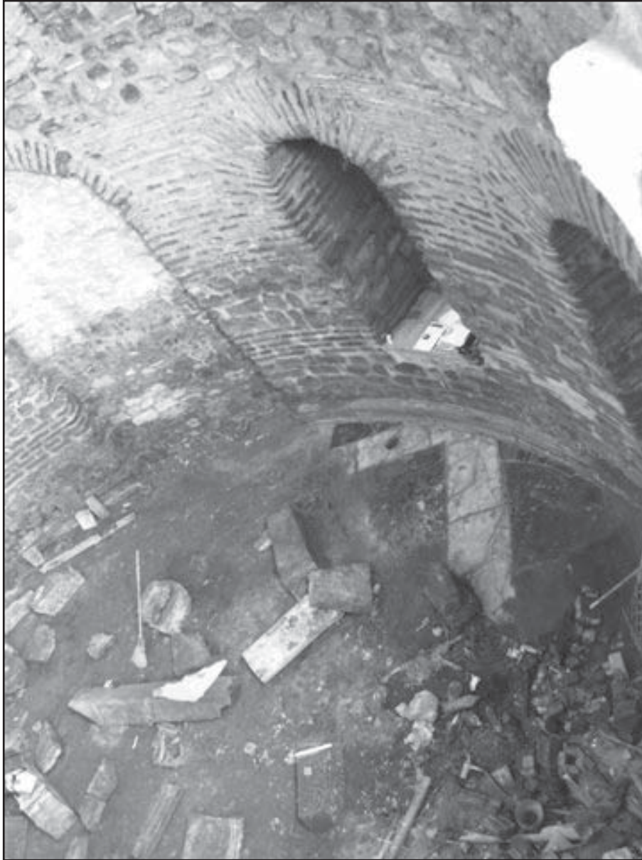
Fig. 4: Skevophylakion, west door, part of the cleaned marble floor, and remains of the marble furnishing
