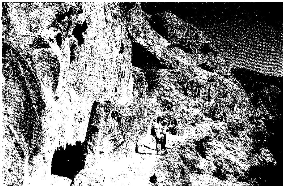
Fig. 6: Rock-cut double path
