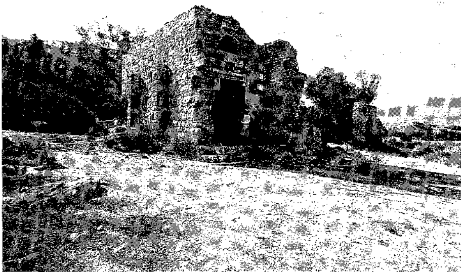
Photo 3: Torba, the “mausoleum” from south-west
