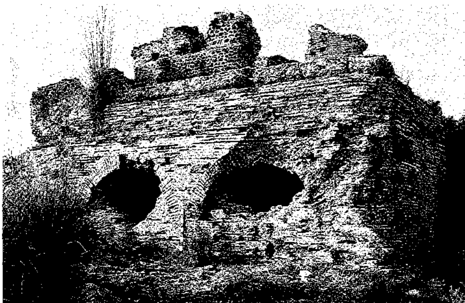
Fig. 14: Building 1 (rectangular chamber at north)
